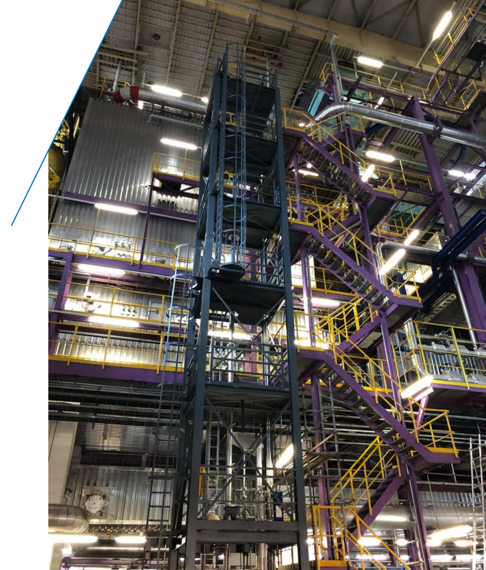
ANDRITZ has supplied its first carbon capture plant to the steel industry. The pilot plant started operating at voestalpine's steel mill in Linz, Austria, in the second quarter of 2023. The plant separates carbon dioxide from the flue gases resulting from iron making using an amine-based process.
